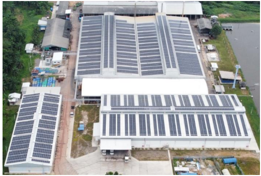
Solar panels at Thai plant
