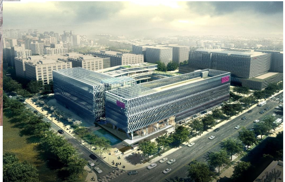
R&D Center Airview Image
